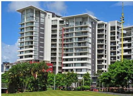
Establishments with Flat Roof
